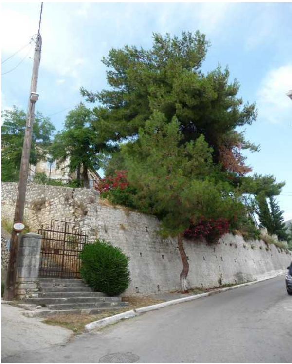
The road further up.
