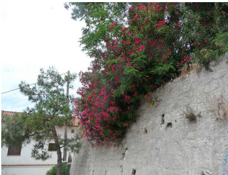
Same cliff with masonry.
