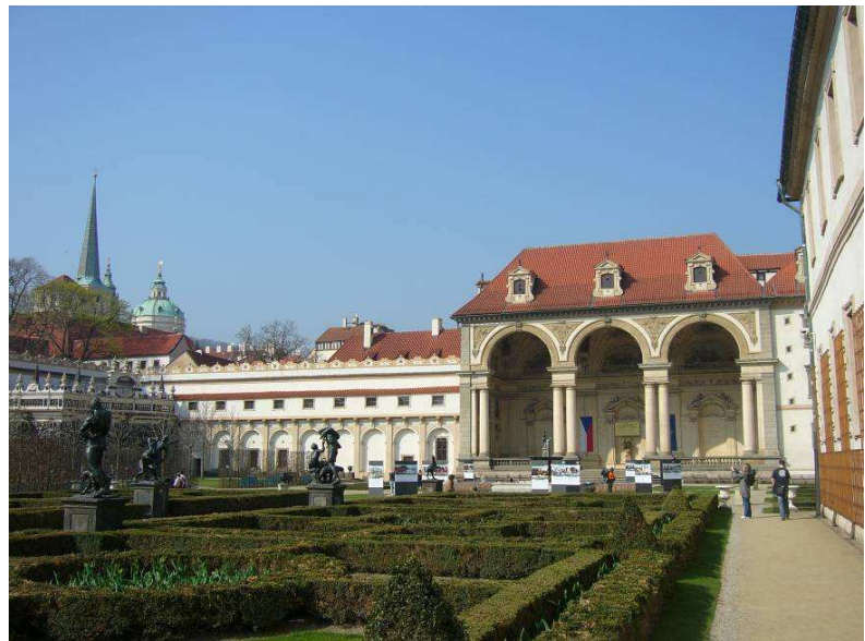
Here we have entered the Wallenstein palace, which was built 1623-29 for the duke of Wallenstein.
