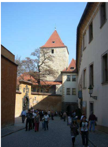
The exit in the north east. The "black" tower is a part of the fortress. It was colored black during a fire in 1541, hence the name.
