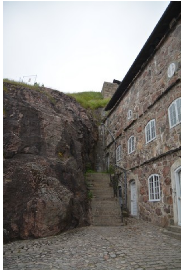
Below eastern curtain wall .
