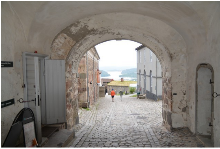
View through eastern curtain wall.
