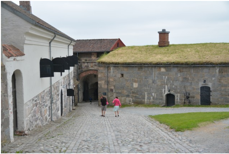
Here we are looking down to western curtain gate .
