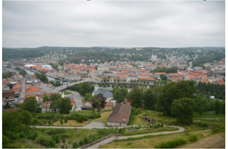
View to the north.
