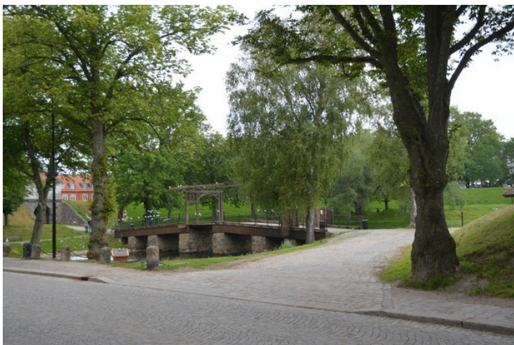
Pedestrian bridge over the moat.
