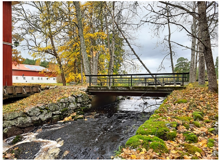
A bridge across the stream.
