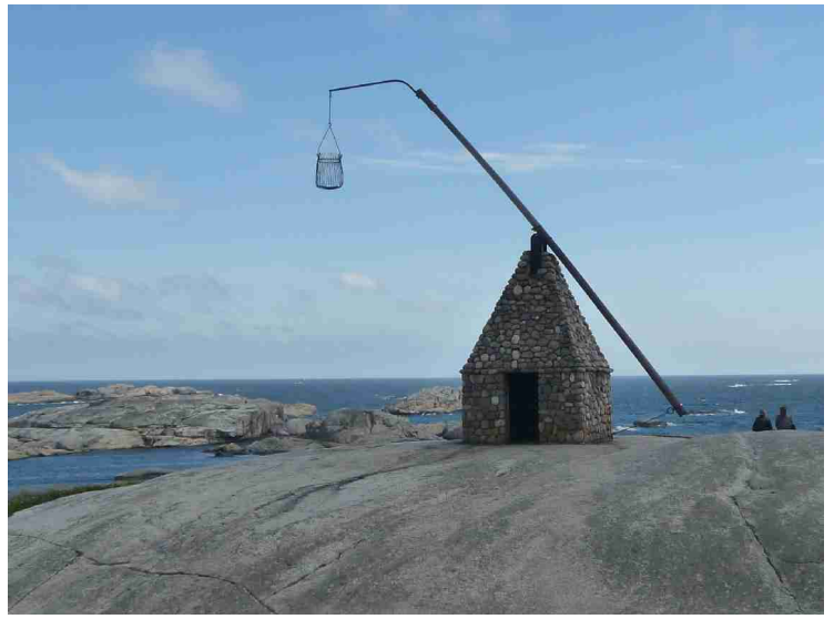
The characteristic tilting light with basket for a coal fire was built as a tourist attraction in 1932.
