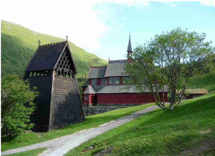
Borgund church is a “long church”, which was built in 1868 and it is still in use.
