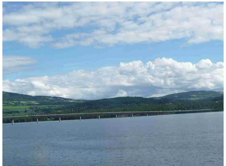
Mjøsbrua (The Mjøsa bridge).
