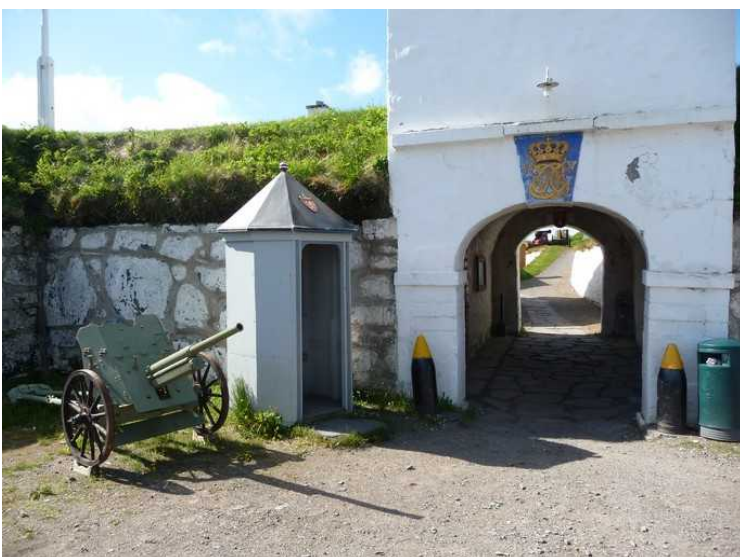
The main gate with the gate building. The gate building was used as a prison in old days.
