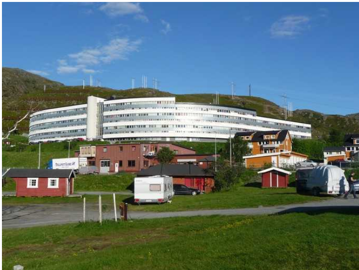
From the camping site we can look up at a large residential block.
