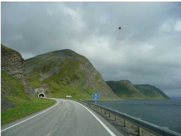
Arriving at the Honningsvåg Tunnel .
