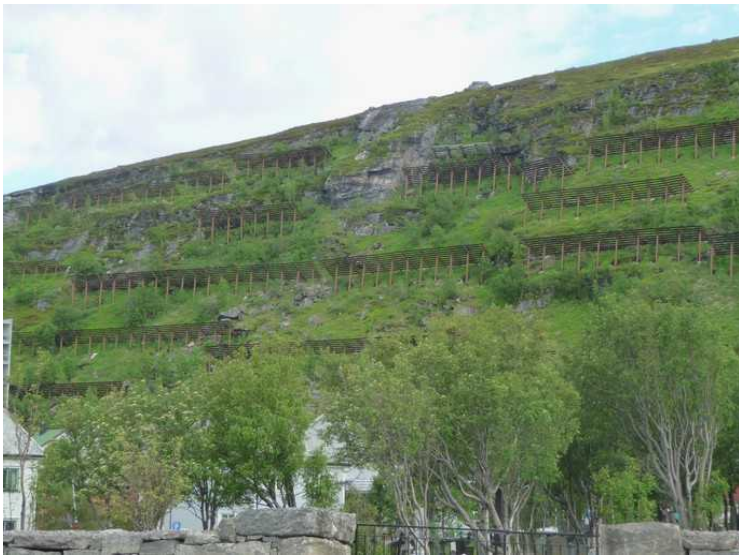
Up in the hillside are made snow barriers to prevent avalanches.
