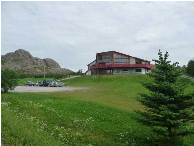
This is the administration building, which is lying on the top of the hill. Here is reception, flats for rent and a large cafe.
