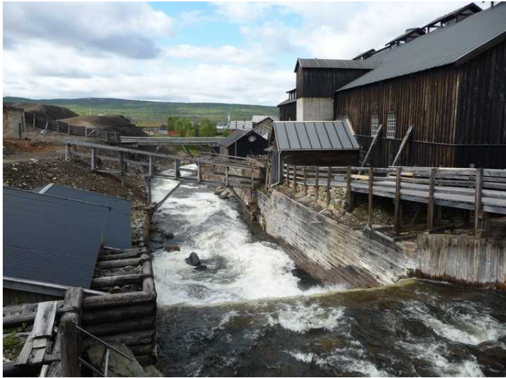
Downstream Hyttelva. The melting hut to the right.
