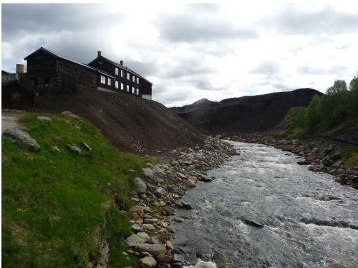
View upstream towards Smeltehytta.
