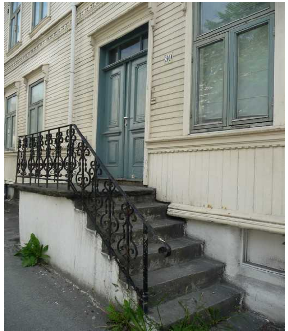
The stairs up into the house.
