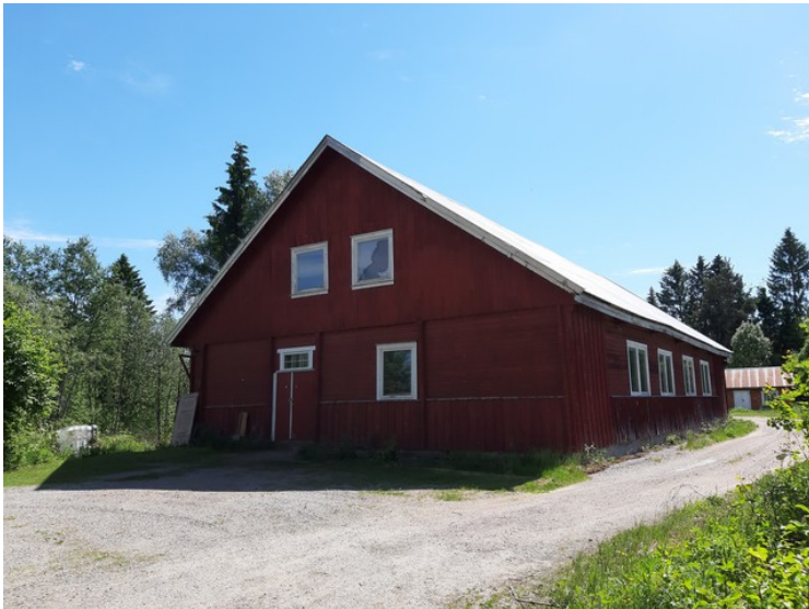
The old spinning mill (carding and spinning). It was built in 1929 and production started in 1920 and continued into the 1950s.
