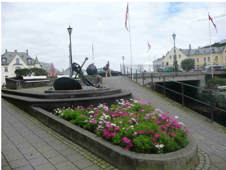
Here Brosundet is on its most narrow. The main road goes over this bridge.
