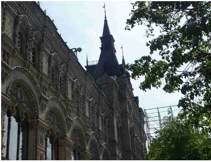
The wall of GUM seen from the restaurant.
