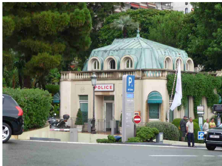
The police station in Monte Carlo.
