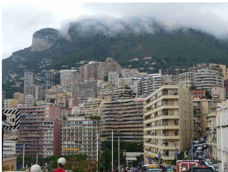
They are building densely and high up in the slope.
