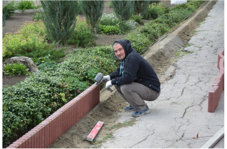
New stones were put in place.
