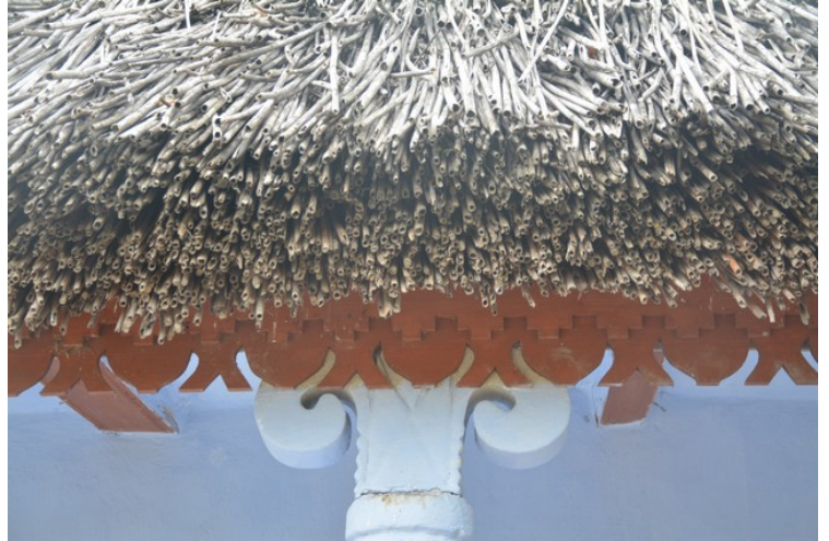
Roofing with reeds.
