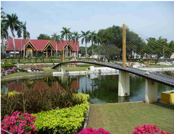
Rama IX bridge, Bangkok, 450 m main span, 6 lanes, finished in 1987. At that time the world's next longest mid-span.
