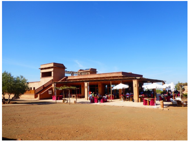
The main building.
