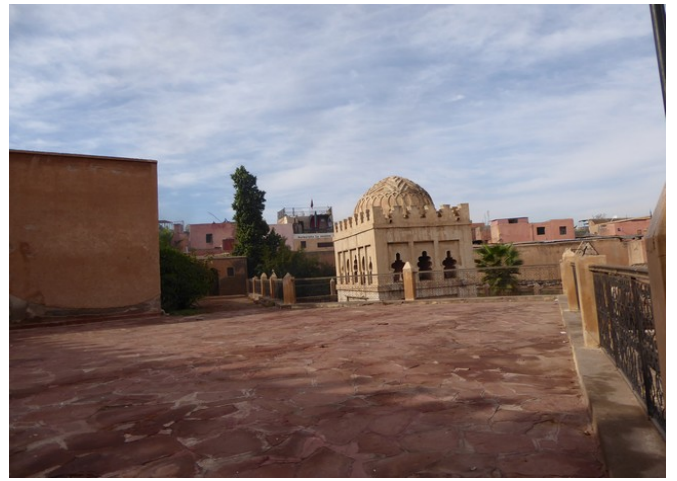
This is the only building remaining in Marrakesh from the Almoravid dynasty . It is called Koubba .
