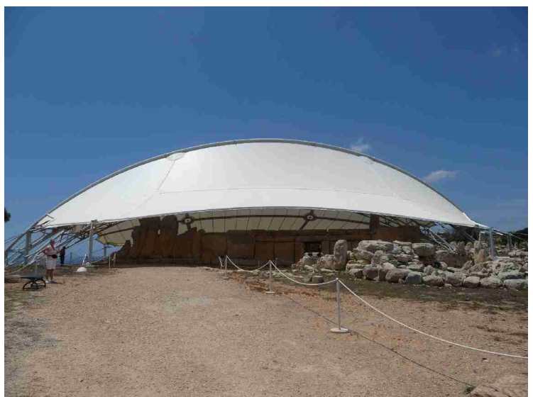
Because of the erosion of the stones, there is put up a tent for protection against the weather. It was finished in 2009.
