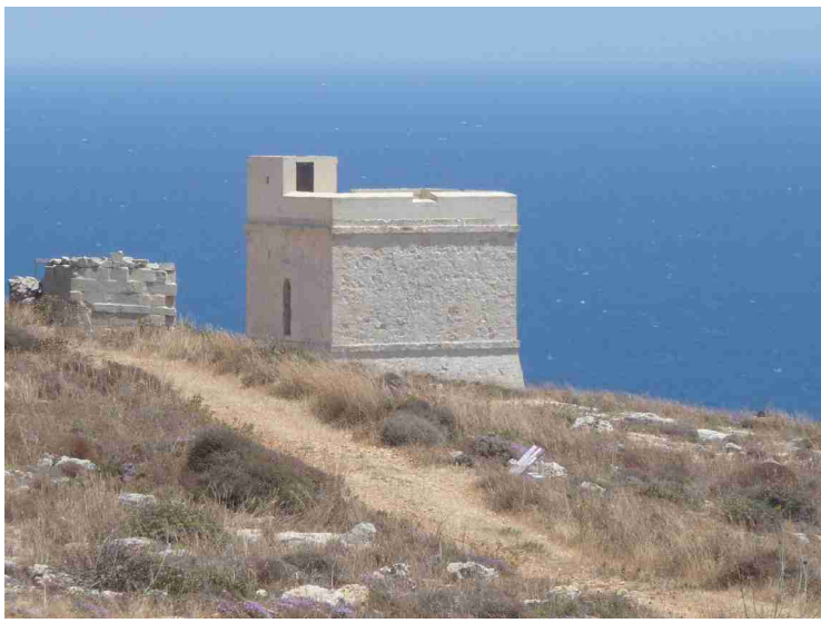
The Namrija tower is one of 13 watch towers that were built in 1658/59 and was a part of the defensive system against enemies.
