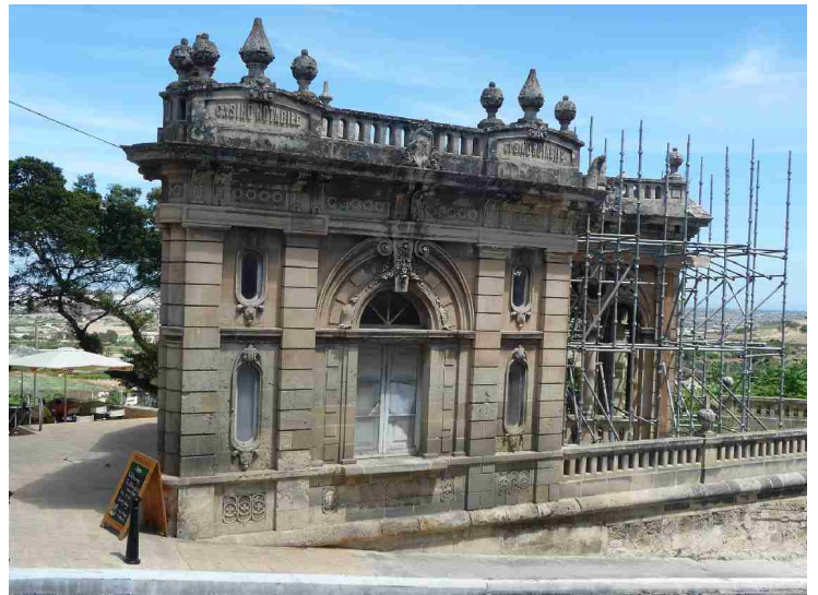
An old mansion. Maintenance work is going on.
