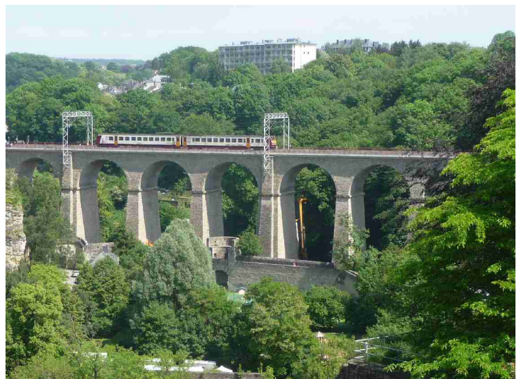
A view to the railway bridge.
