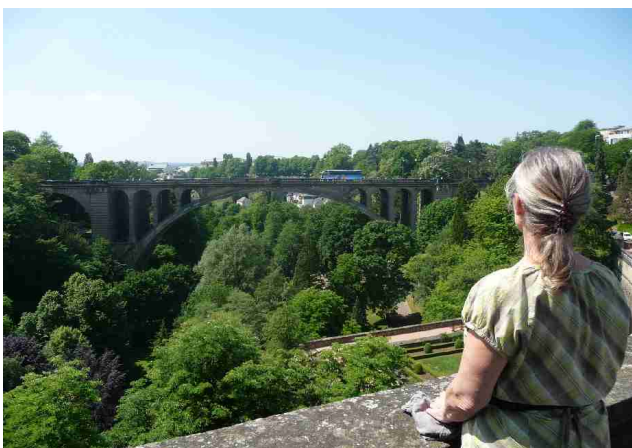
Anne Berit is looking across the Petrusse valley to the Adolphe bridge . It was built 1900-1903 and had at that time the worlds longest span for a stone bridge.
