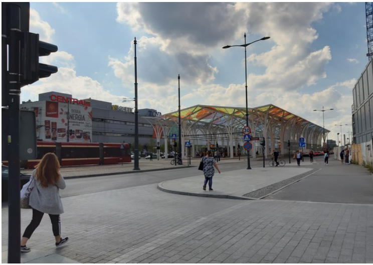
Here we look towards Dworzec tram station , which is the hub of two tram lines, north-south and east-west. It opened in 2015.
