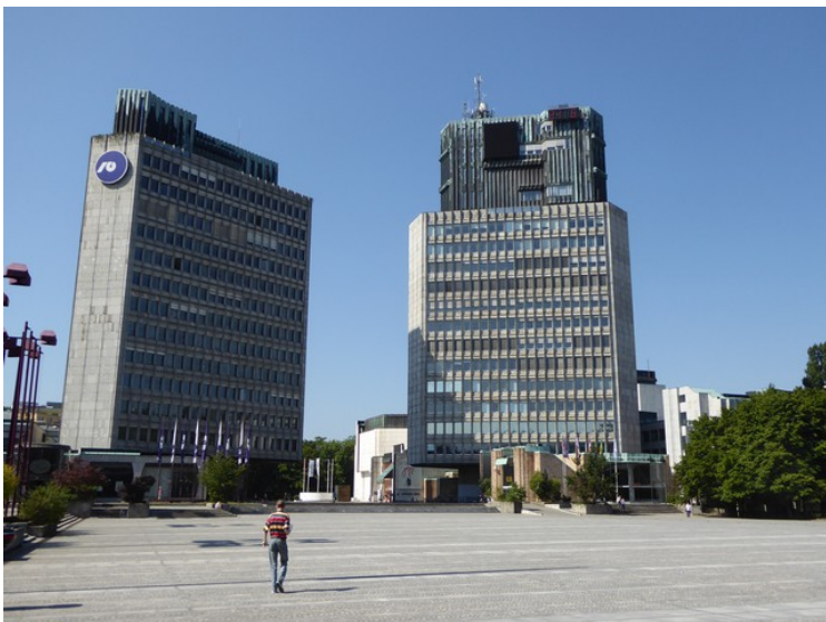
This is Trg Republike Square , which lies in front of the Parliament building.
