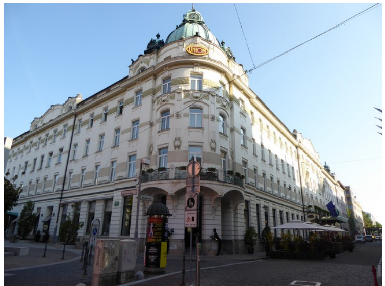
The following day we went down to the center past Grand Hotel Union . Large building.
