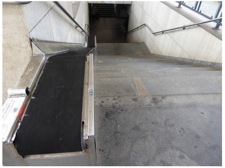
This is a heavy luggage conveyor. Instead of dragging the luggage up the stairs, the luggage is put on the belt and it starts to go. Easy!
