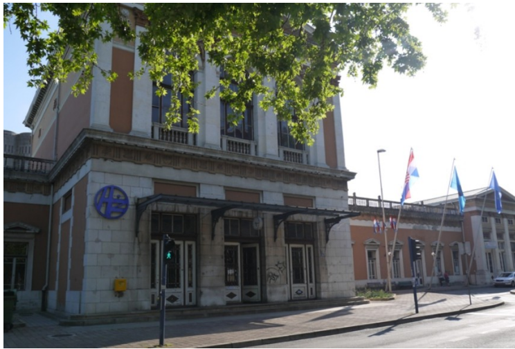
The railway station in Rijeka. The building is quite big, but it seemed quite dilapidated.
