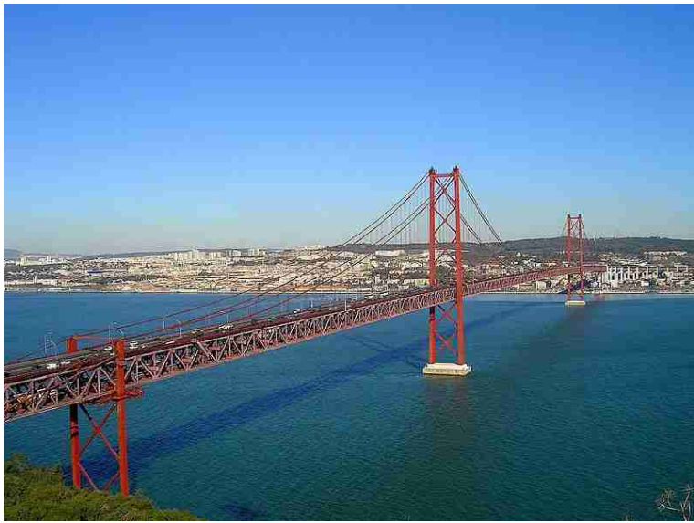
We went over the 25 April bridge .
