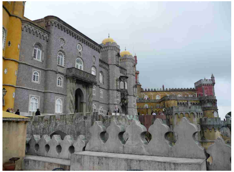
In the grey section is the biggest hall, the ambassador hall, which was used for receptions. The front is covered with ceramic tiles.
