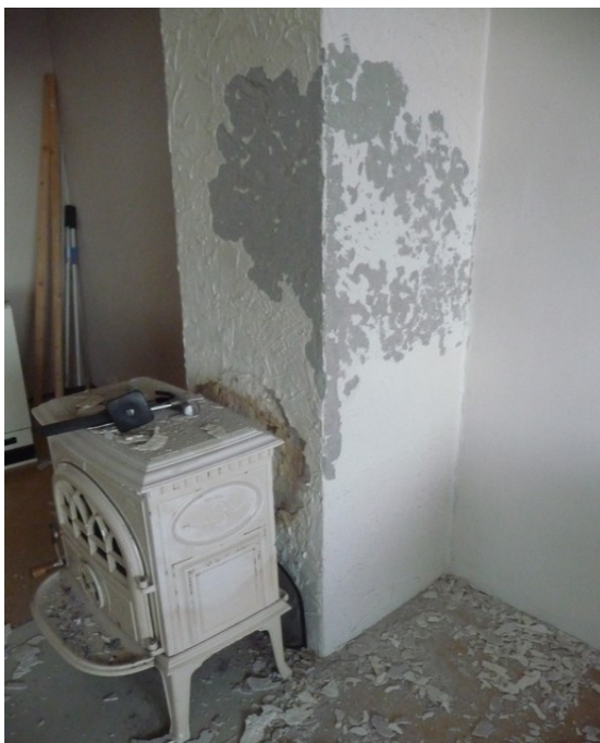
The chimney was smeared in with a thick layer of texture paint. It was flaky and not very nicely, so I spent three days to remove the layer.
