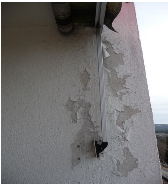
This is out on the balcony. On the walls the paint is peeling and the railing is smeared with the same texture paint as there was on the chimney. The railing is ruined. It was originally fine anodized aluminum. We checked the possibility to get new railings in the original version, but it had cost nearly NOK 30 000. Too expensive.
