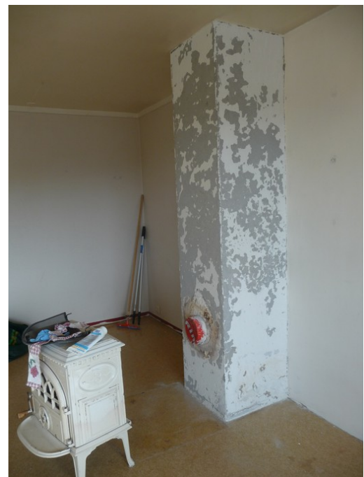
The chimney was smeared in with a thick layer of texture paint. It was flaky and not very nicely, so I spent three days to remove the layer.
