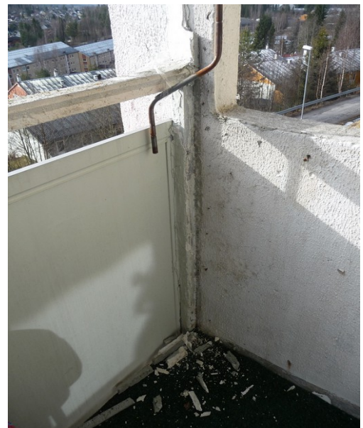
This is out on the balcony. On the walls the paint is peeling and the railing is smeared with the same texture paint as there was on the chimney. The railing is ruined. It was originally fine anodized aluminum. We checked the possibility to get new railings in the original version, but it had cost nearly NOK 30 000. Too expensive.
