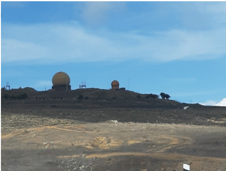
This is the installation of Escuadron de Vigilancia Aerea. It is an air surveillance station.
