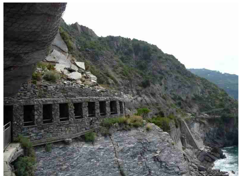
The path is partly cut out of the mountain and supported by concrete
