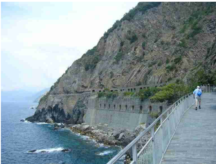
The path is partly cut out of the mountain and supported by concrete
