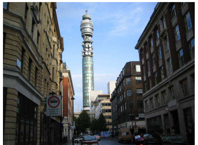
Here we went past the tower of British Telecom. The building started in 1961 and it was opened in 1965. It should have been 111m high, but it has sunk 53m afterwards. It had a rotating restaurant on the top, but it is now closed for the public.
