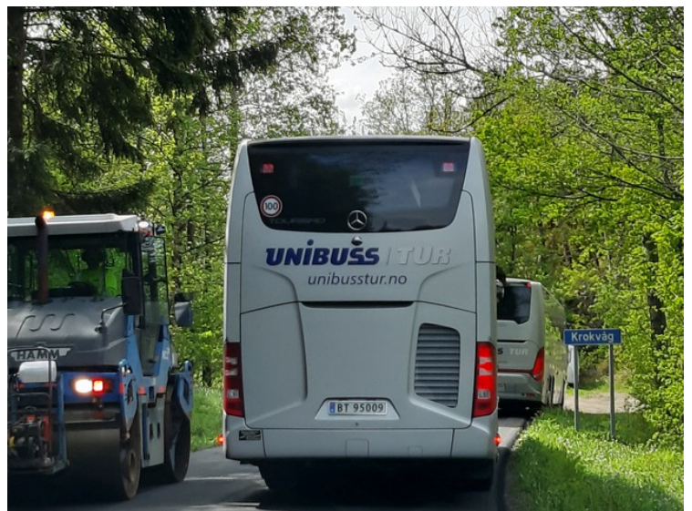
In Krokvåg, just before Tvedestrand, we are behind two tour buses that had to wait due to road work.
