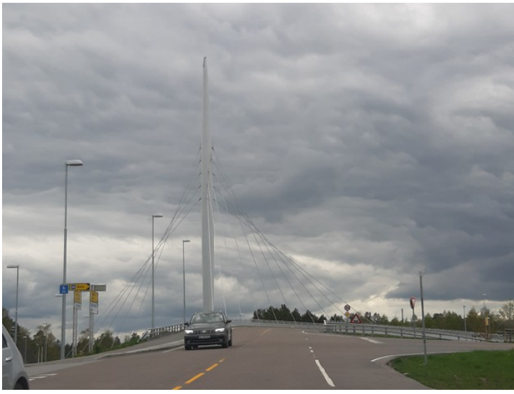
Here we come to Ørje. We will drive on this bridge that crosses the E18. It is called Norgespporten Bru.
