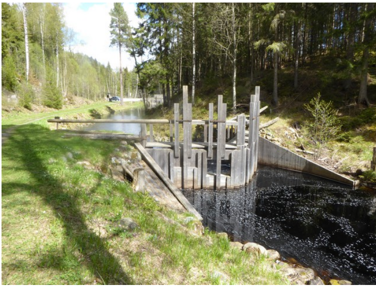
The lock gate seen from above.
