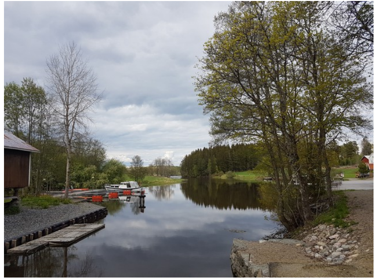
View north from the lock chamber.
