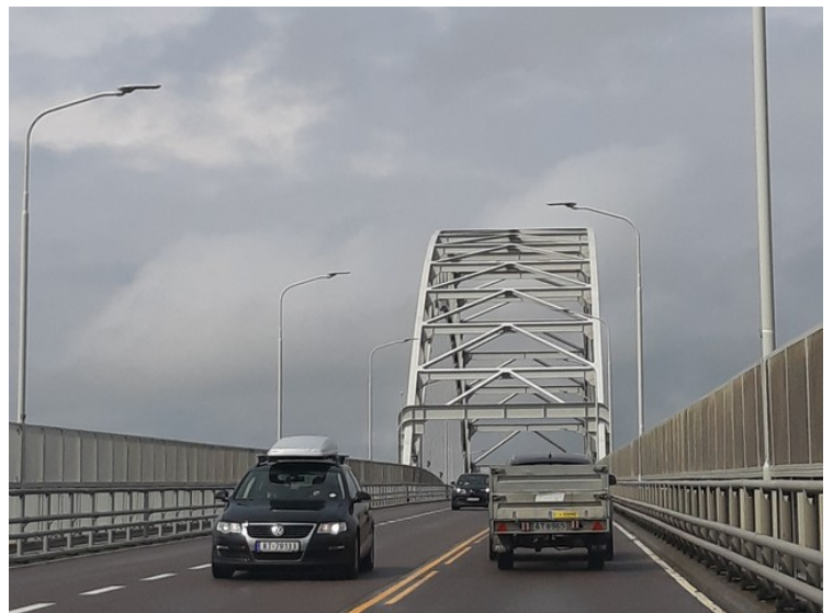
This is just before we get to Fredrikstad , Fredrikstad Bridge .
