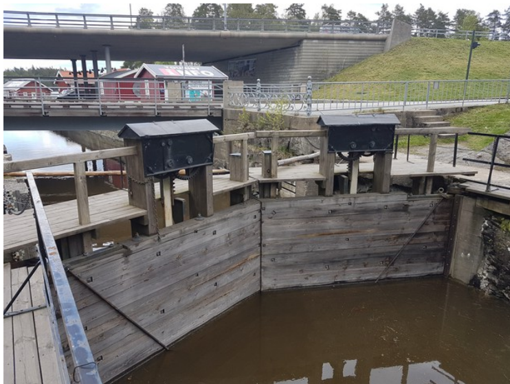
This is the upper lock gate.
