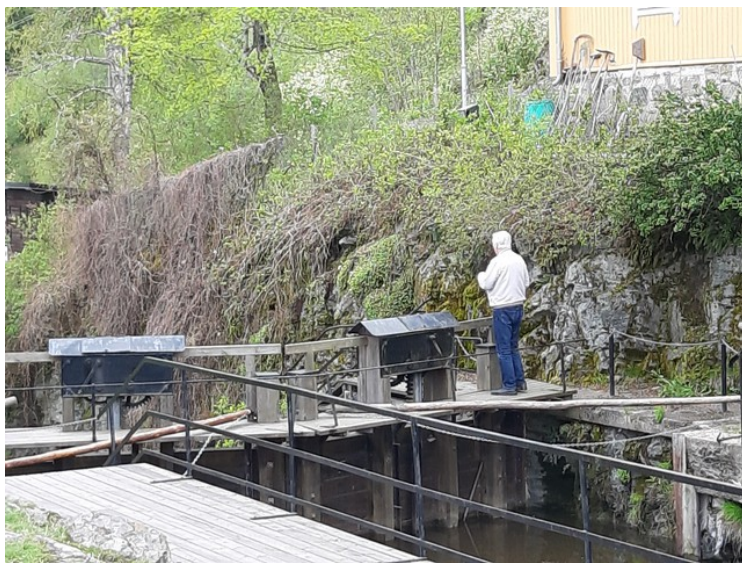
I was most interested in the canal. Here I will check if the locks are in order.
