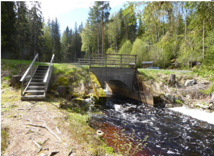
The lock and the gate seen from below.
