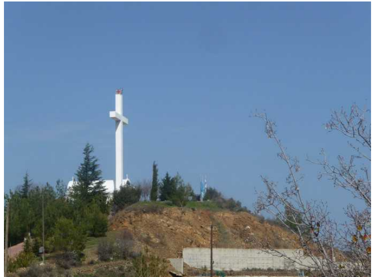
On Fidkias peak right at Pedoulas is erected a small church and a 25m high cross, The holy cross , in honor of those killed in the Balkan wars of 1912-13.
