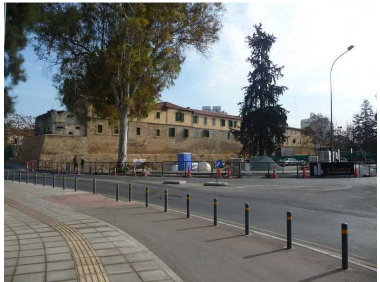
Here is another part of the wall seen from the outside.
