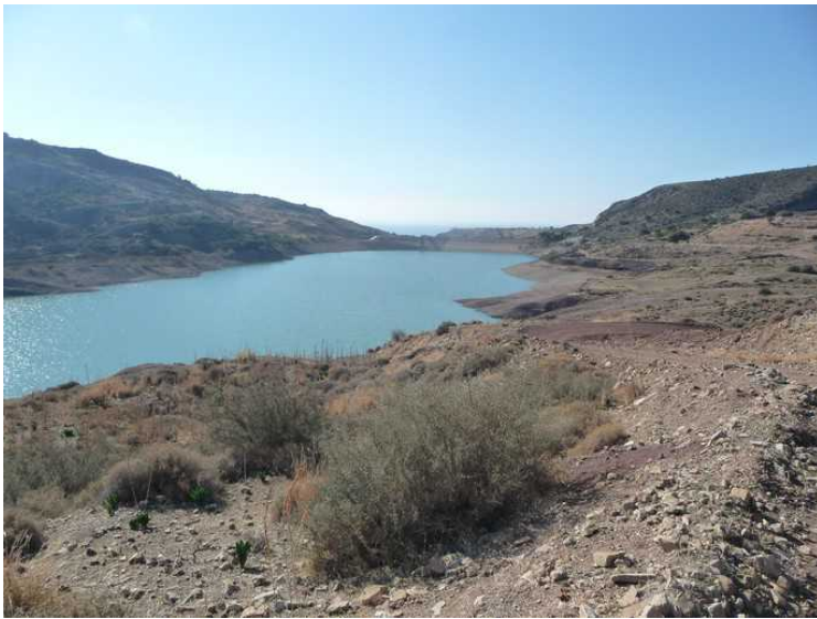
Here we are at the end of the lake and are shooting the picture outwards in the direction of the dam. The Mediterranean Sea in background.
