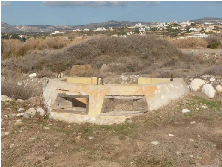
This is a bunker, probably from the liberation war 1955-59.
