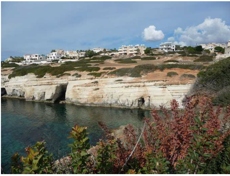
Cliff caves in the steep slope.
