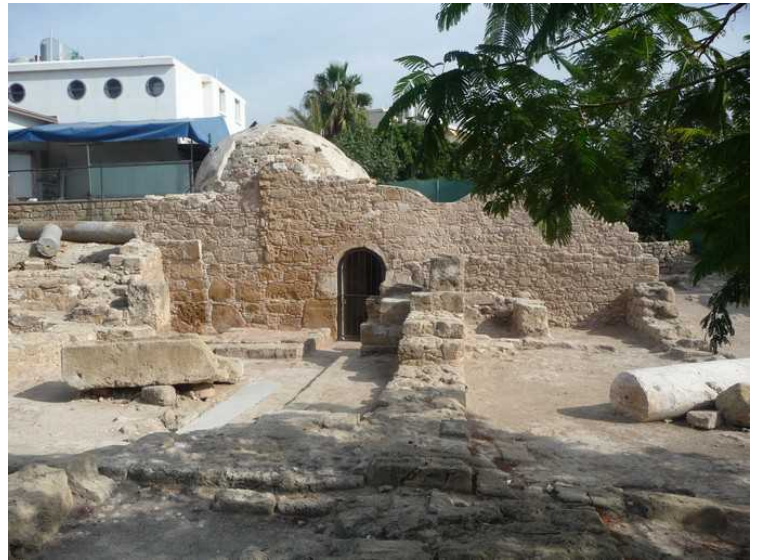
The main building is being restored. There has been granted funding from the EU. Newspaper article .
