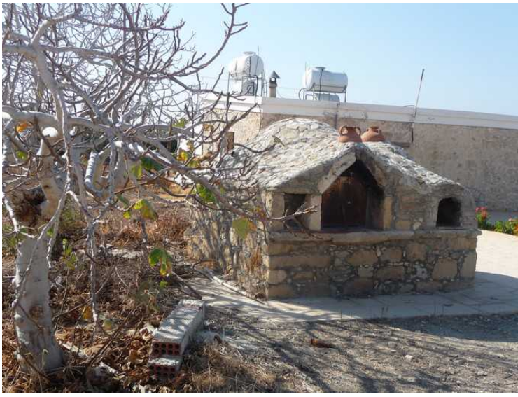
What this little building used to, we do not know. We think that it had been used as a hostel for pilgrims.
