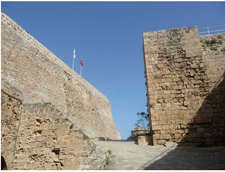
On the way to the north west tower.
