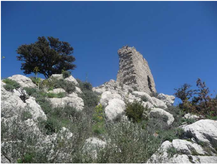
The upper tower.
