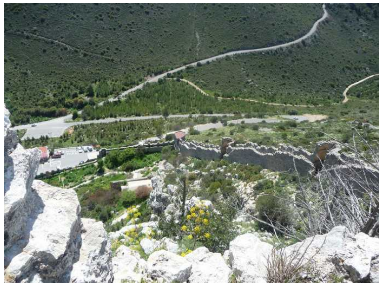
View down along the wall and down to the parking lot.
