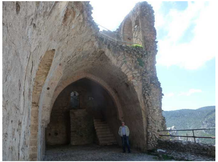
Inside. The roof is gone.
