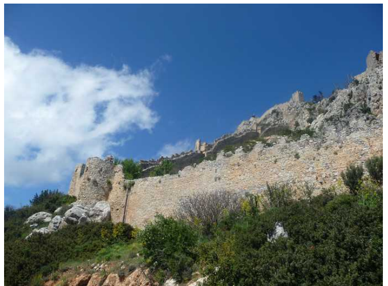
Here we see some of the lower walls.
