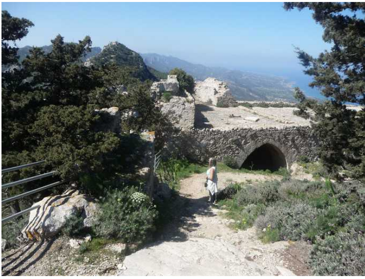
The vaulted chambers.
