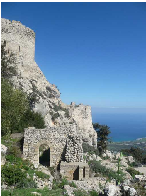
At the top we see the horseshoe-shaped tower and below it a Byzantine tower.
