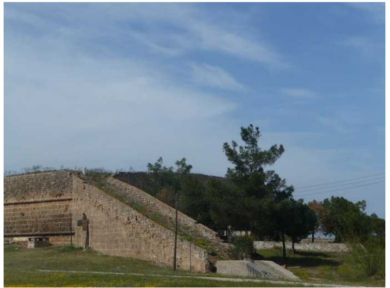
A part of the walls of the Martinengo Bastion .
