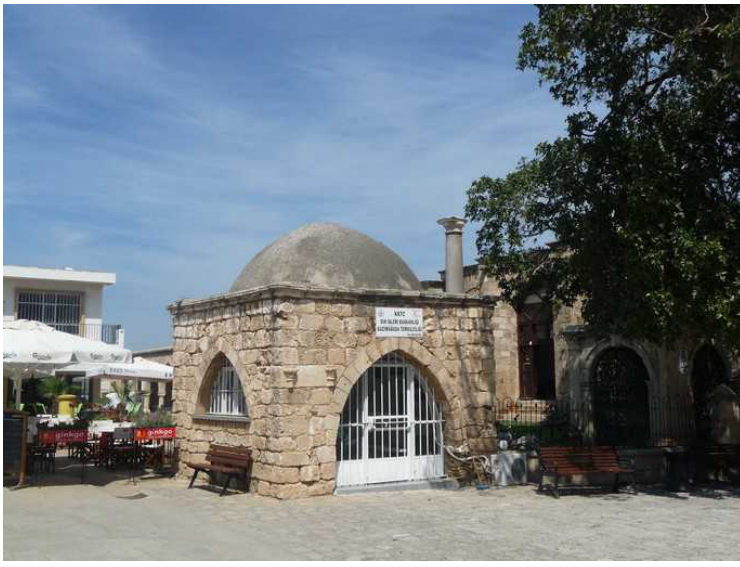
A small building next to the mosque.
