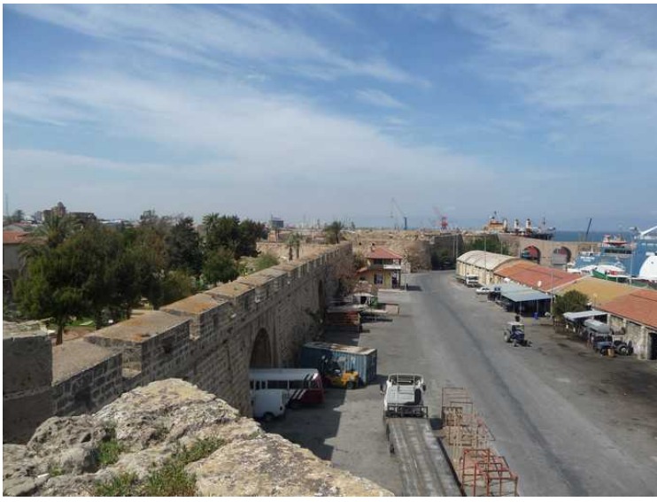
Here we are on Othello's Tower and looking north on the outside of the wall.
