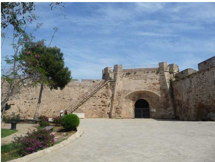
The old town of Famagusta is surrounded by a fortified wall that encircles the entire city. Link . Here we come to the part closest to the port.
