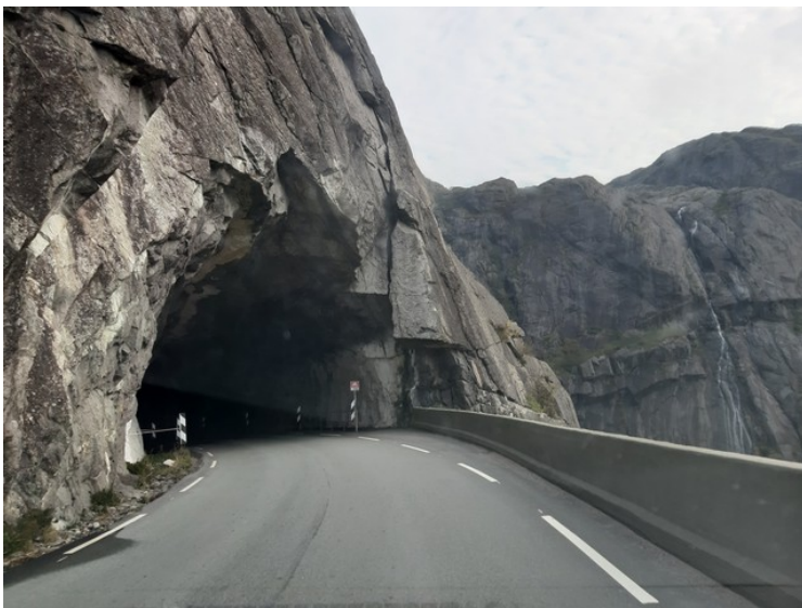
On the way further down we have to go through a tunnel.
