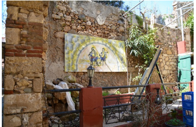
This place was a restaurant when I was here the last time in 1991. It is evident that it was shut down many years ago.
