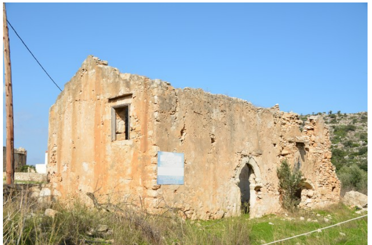
There are old ruin houses around the church.
