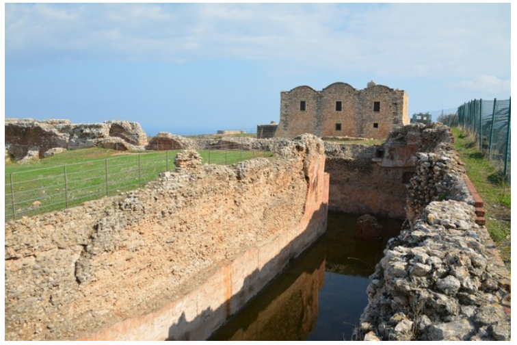
After that we drove back to ancient Aptera. Right at the entrance we see one of cisterns in the area.
