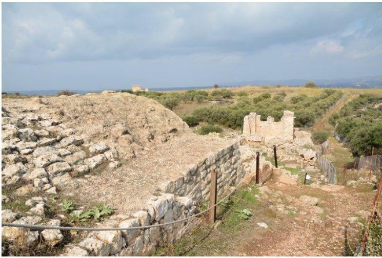
The roof of cisterns below the monastery.
