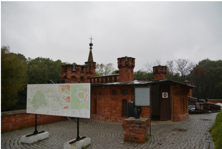
Here we have moved to the top of the entrance building.
