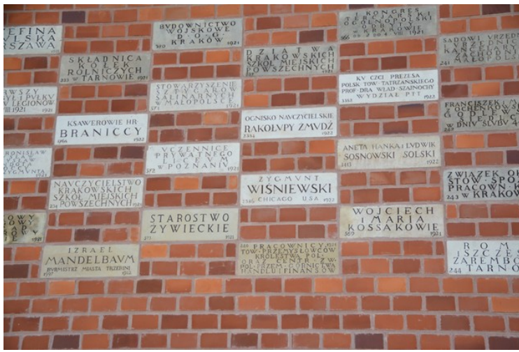
In the early 1900s there was made major maintenance work on Wawel Hill. The money needed for this was done by gathering. All those who gave any amount got their name on a brick.
