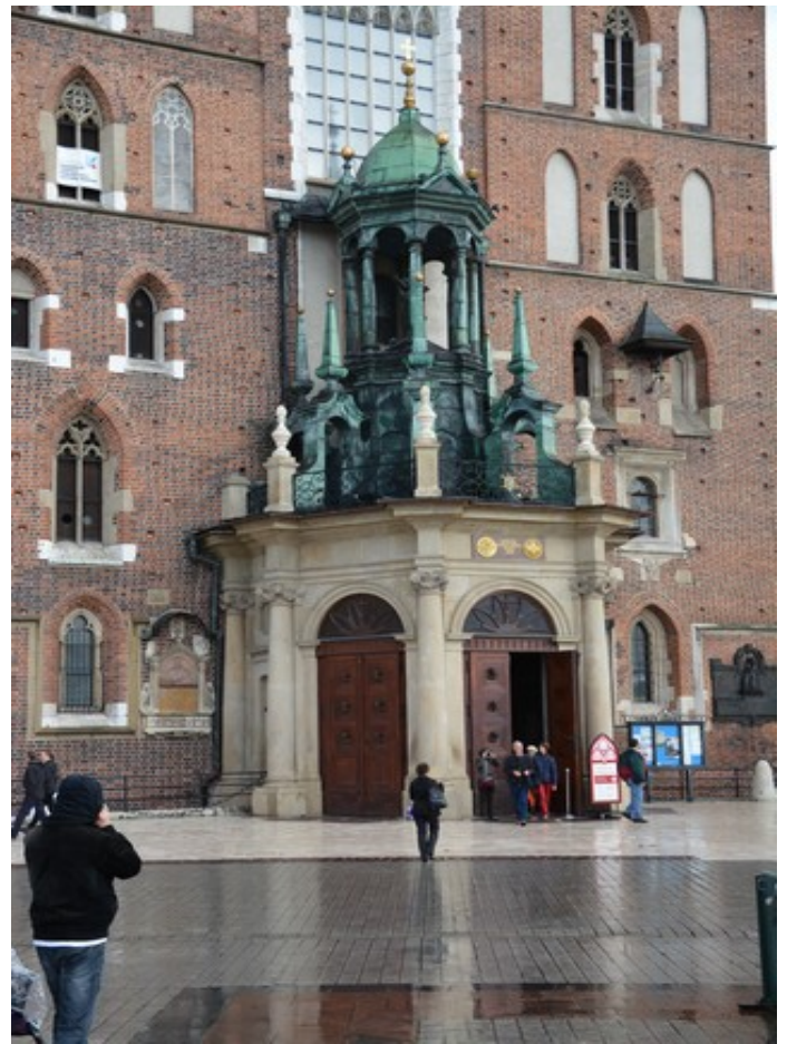
The front of St. Mary's Church.
