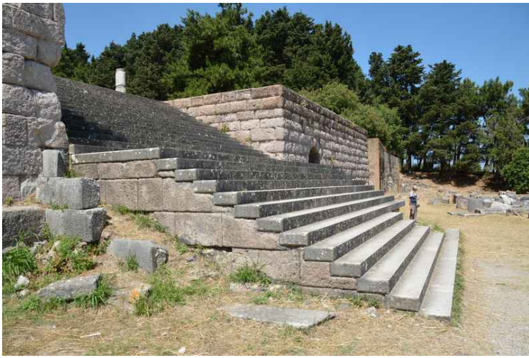
The stairs up to the 3rd level.
