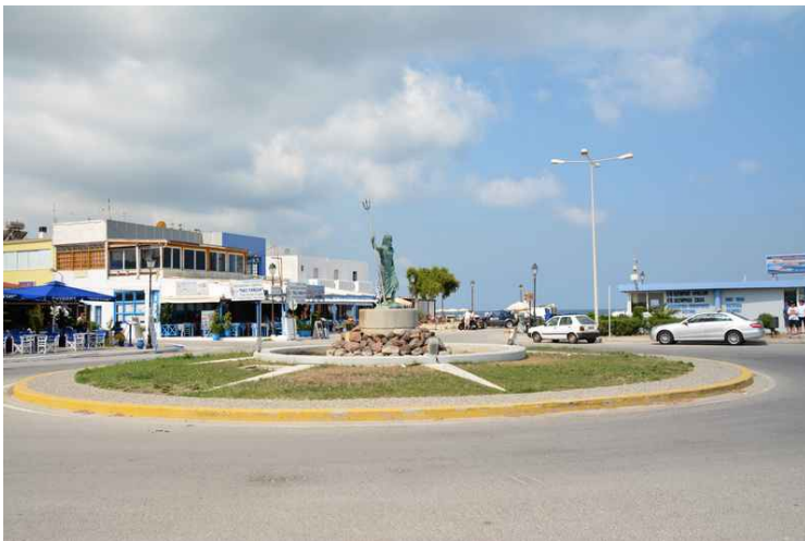
There is a large roundabout with exits to the east, to the pier, to the beach and into the town center.
