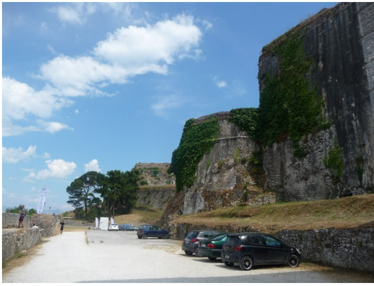
Walls on the north side.
